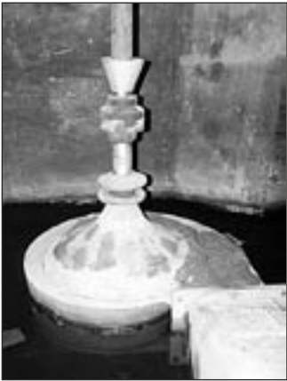
The mill has a Ridgeway and Sons Scroll Turbine
