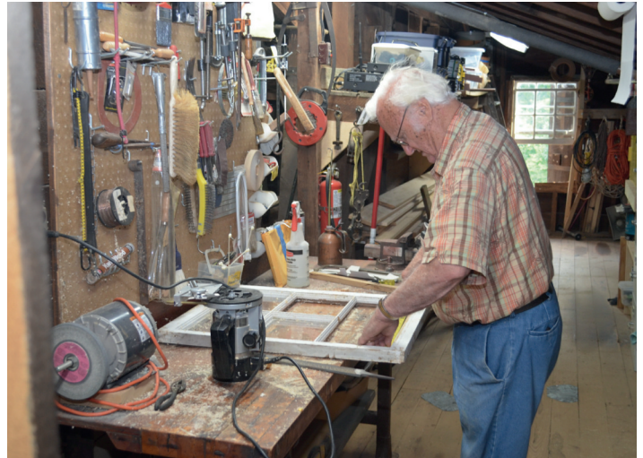
Clarence Klauer (Dick's brother) is repairing a window that had a mullion broken out of it.
