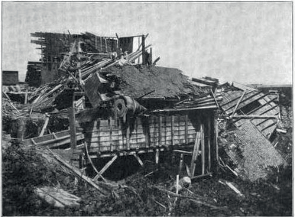
WILSONVILLE, NEB., ROLLER MILLS, AFTER THE BOILER EXPLODED.
