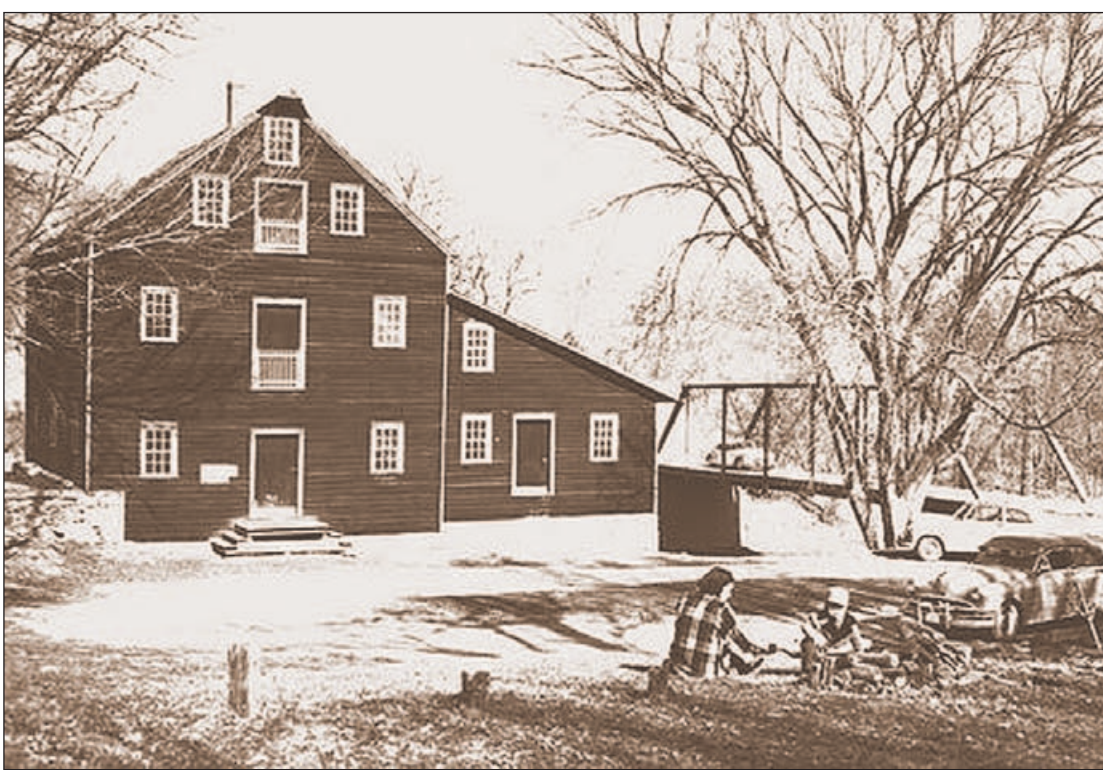
The Pine Creek Grist Mill, sometime during the late 1950s.
