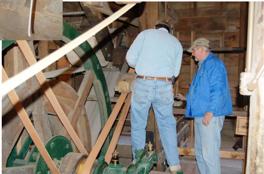
Scott Gibbs and Jerry Kieth installing the new idler mount for the water pump drive belt.
