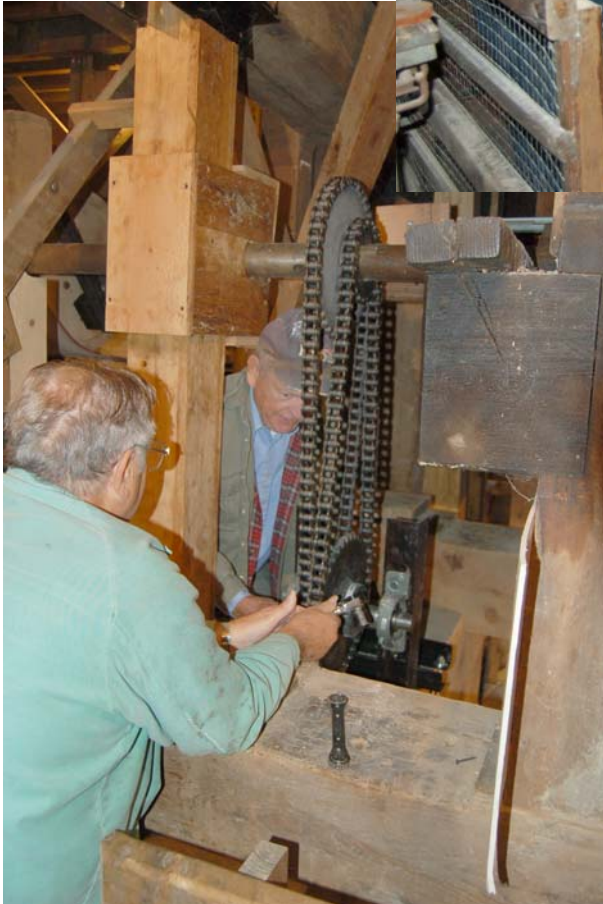
Scott Gibbs and Jerry Kieth installing the new idler mount for the water pump drive belt.
